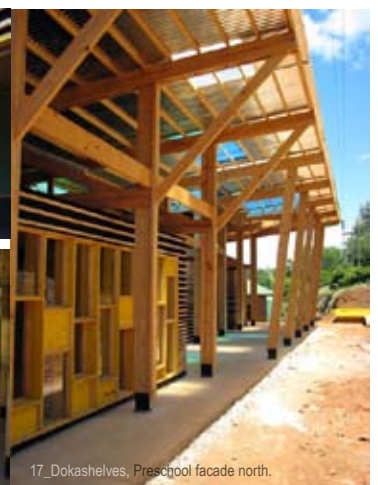
17_Dokashelves, Preschool facade north.
