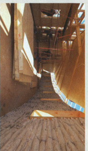
Box frame windows in a wall of earth-filled bags.
