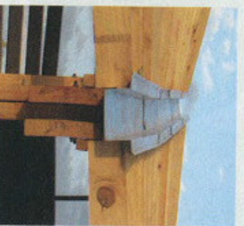
Metal gutter between bays.
